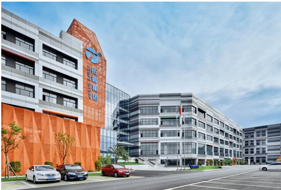
2023-07-17-Tuopu-3.jpg Tuopu headquarter in Ningbo
