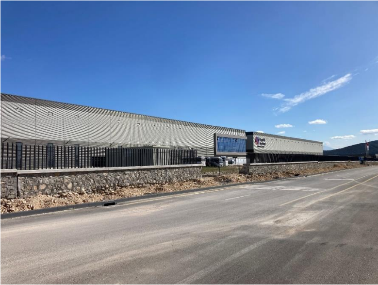
LiCON-Success-Story-Celikform-2.jpg Celikform Greenfield plant at Technosab site
